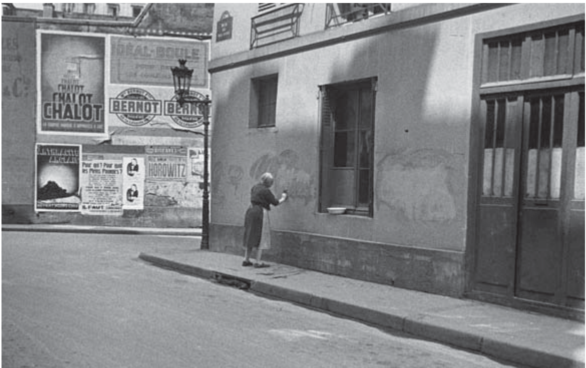
Gisèle Freund, 'Cleaning of a house facade, Paris', 1935.
